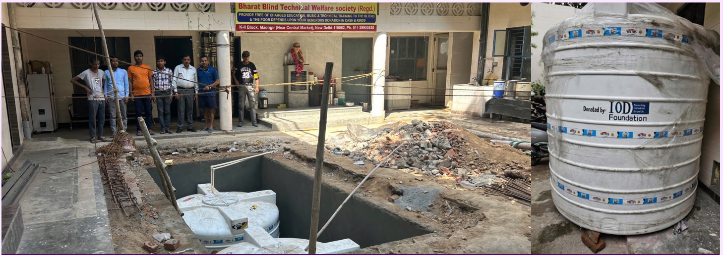
Installation of the Water Tanks
